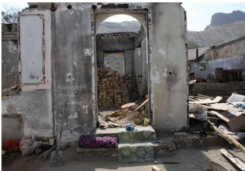
Damaged house, Osh region
