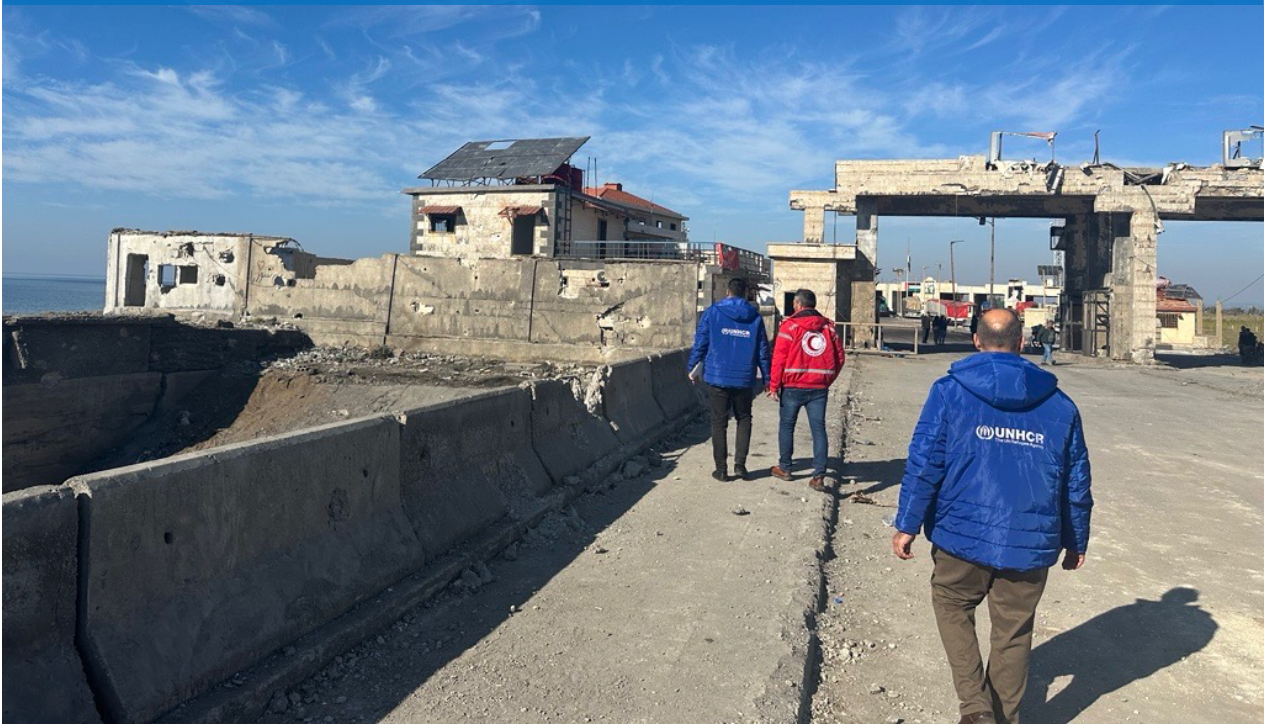
UNHCR and its partners supporting those crossing the recently reopened Al-Arida border crossing, still visibly damaged on 3 December | ©UNHCR Syria
