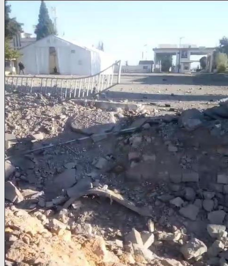
Damage at Joussieh border crossing | ©SARC
