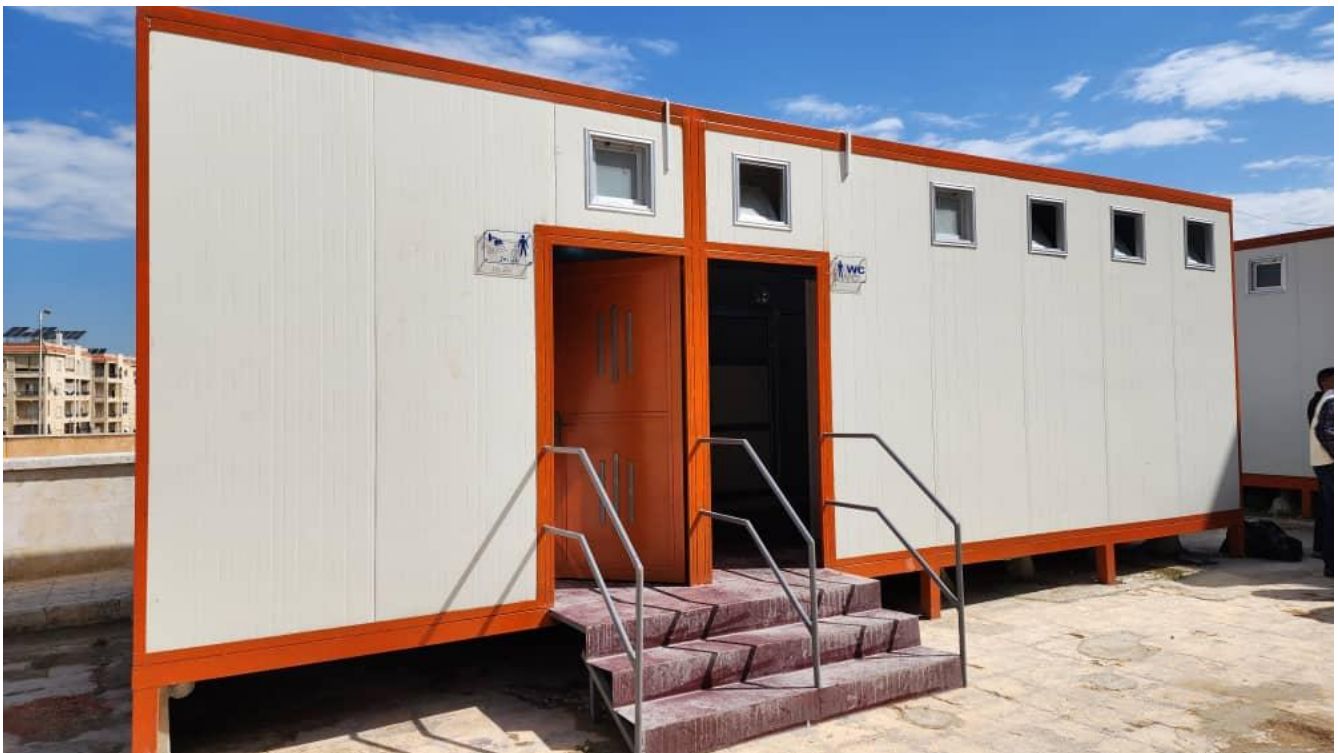
UNHCR and partners conduct adaptation works in collective shelters of Aleppo Governorate, including gender-segregated restrooms, ensuring that protection standards are in place. Photo: ©UNHCR/Z. Ayoubi
