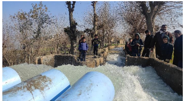
The irrigation system repaired by UNHCR in Deir-ez-Zor. ©UNHCR/M. Abssi
