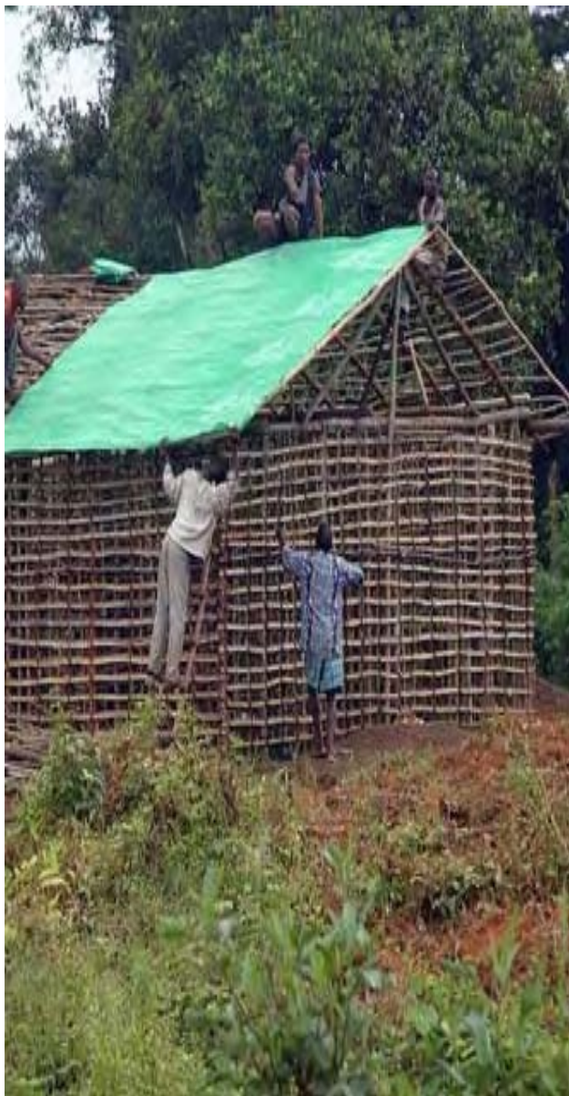
Reconstruction in progress in Kombohahun Town, Kolahun district, Liberia. / UNHCR
