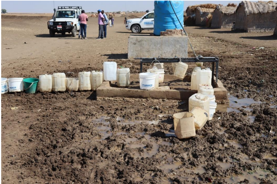
Figure 2: Lack of drainage at water tap stands lead to jerricans standing in a mud pool.
