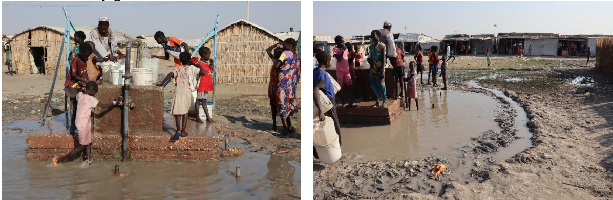
Figure 5: Swamped water points; proper drainage, which could lead to formal reuse, would be very beneficial.
