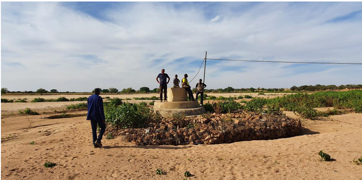
Figure 6. This well protection in Mile already captures most of the logic behind the solution.
