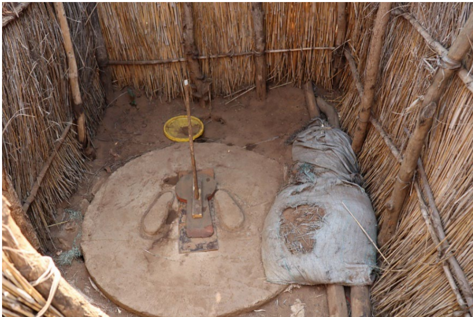
Figure 8: SanPlat with movable lid, Zambia
