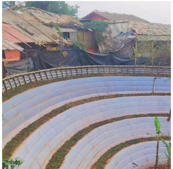
Geo-tube terracing. Inter-Sector Coordination Group, 2022
