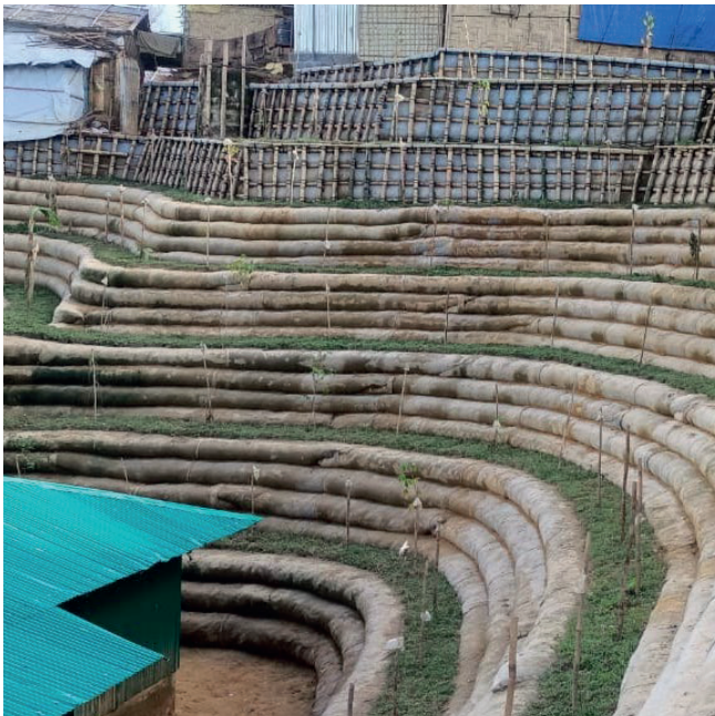
Geo-tube terracing. Inter-Sector Coordination Group, 2022
