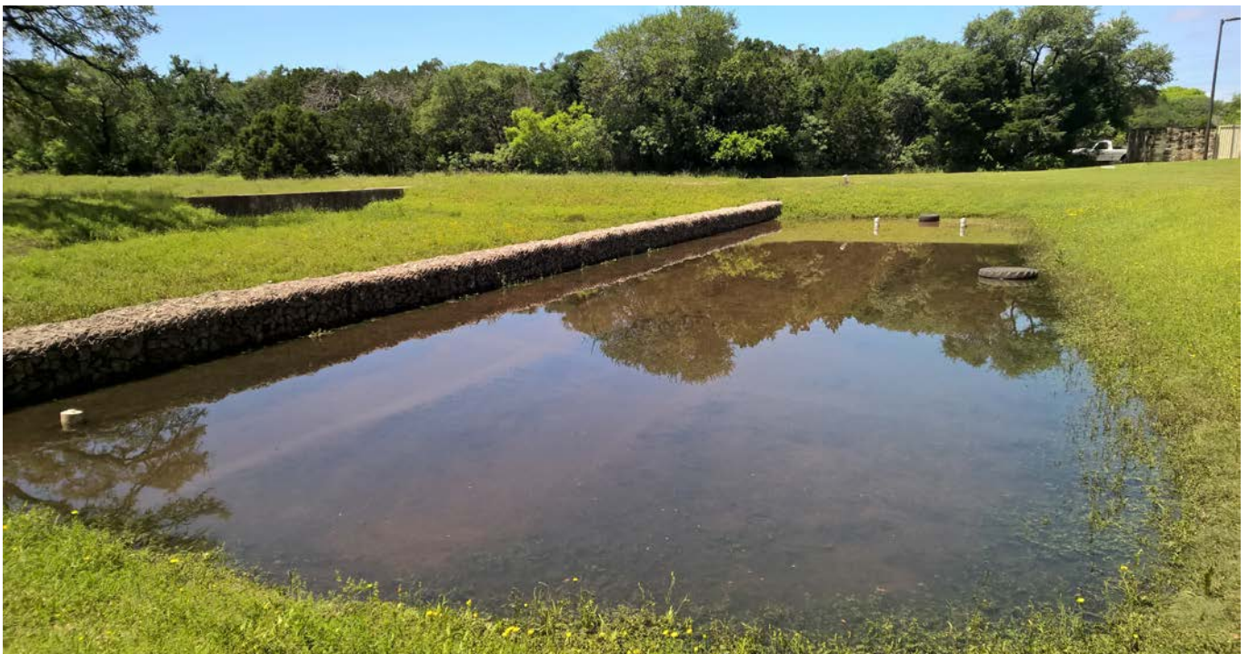
Partially filled retention pond
