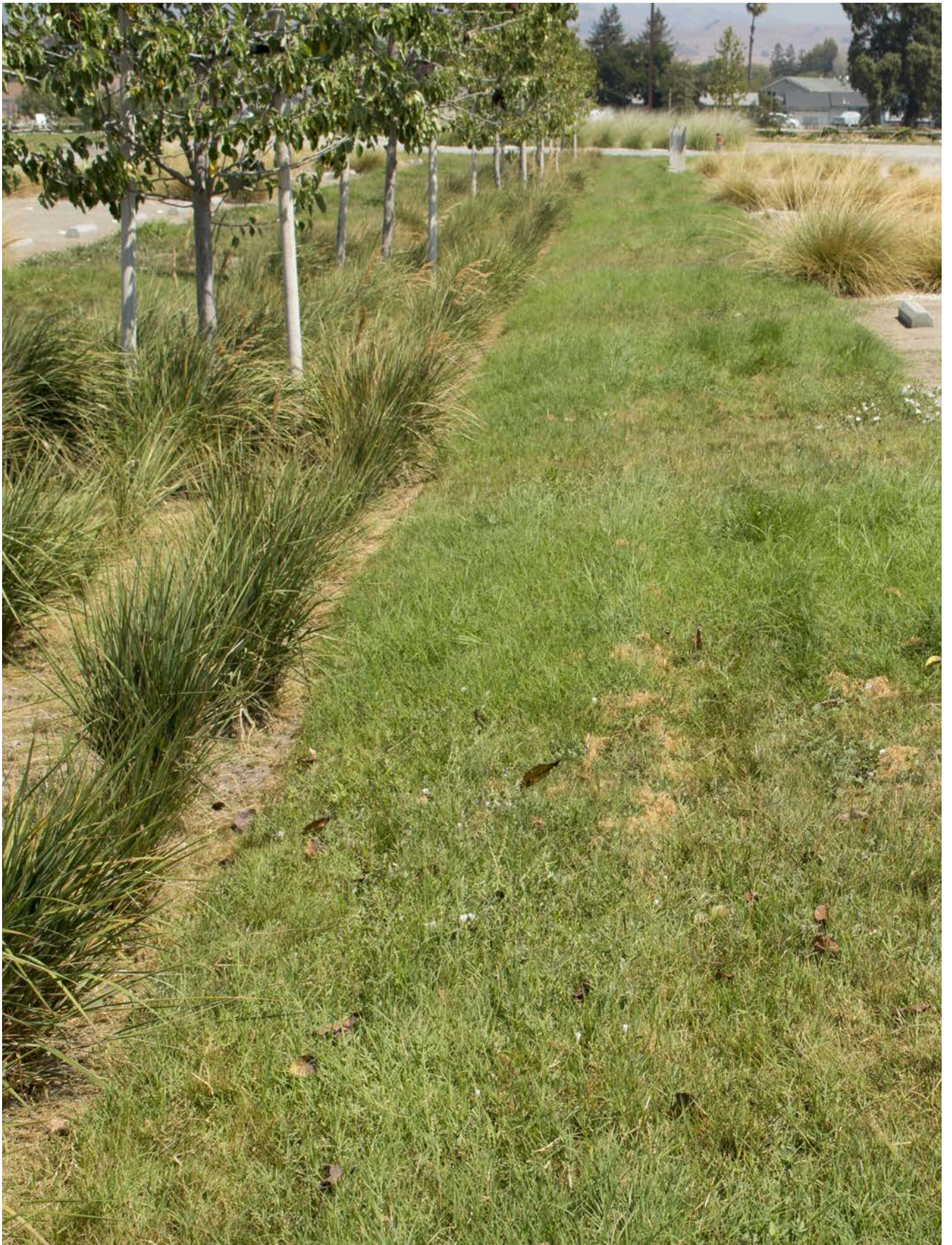
A drainage swale integrated with a carpark
