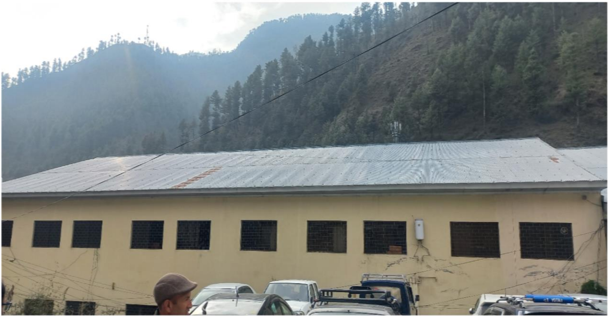
Solar PV (Shutter Rooftop)
