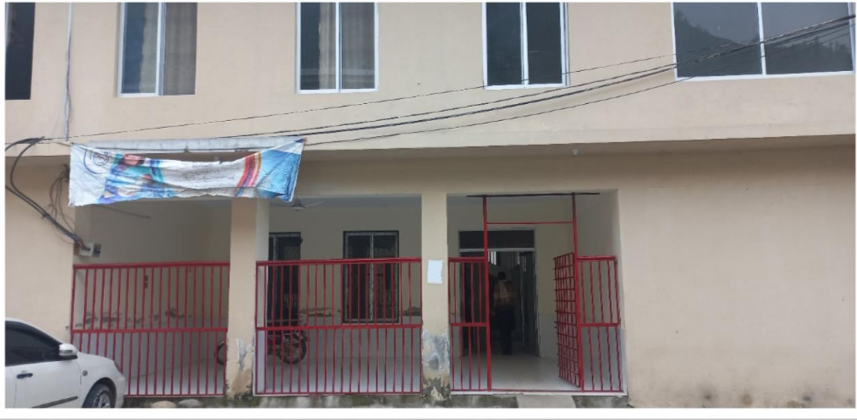
Solar PV (Shutter Rooftop at X-Ray Building)
