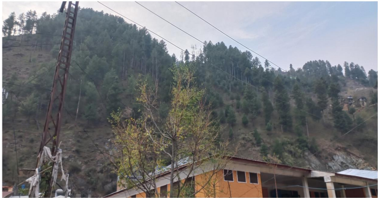
Solar PV (Shutter Rooftop at Gynae Block)
