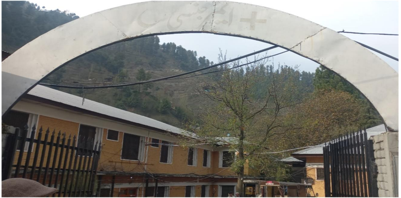
Solar PV (Shutter Rooftop at PEADS Ward)
