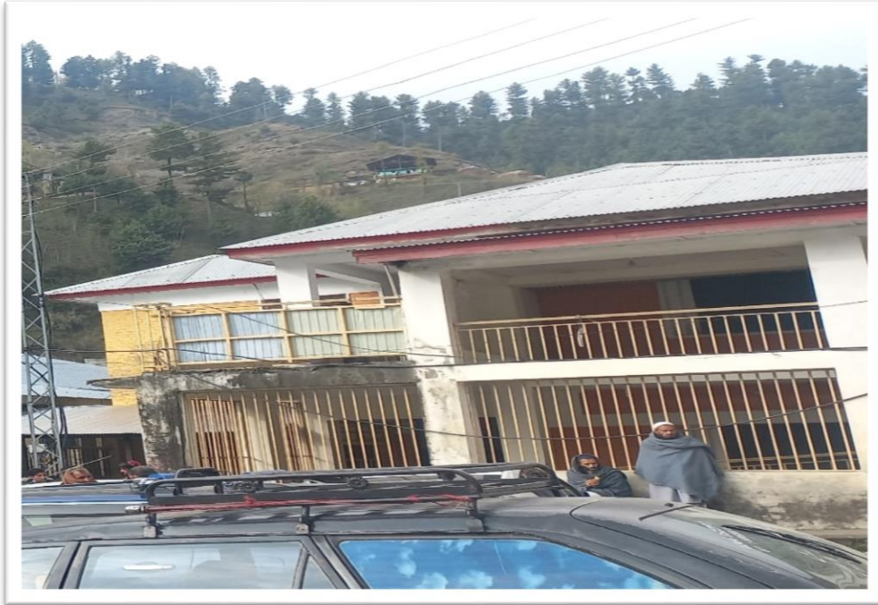
Solar PV (Shutter Rooftop of Wards)
