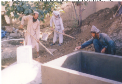
Constructing a biogas plant
