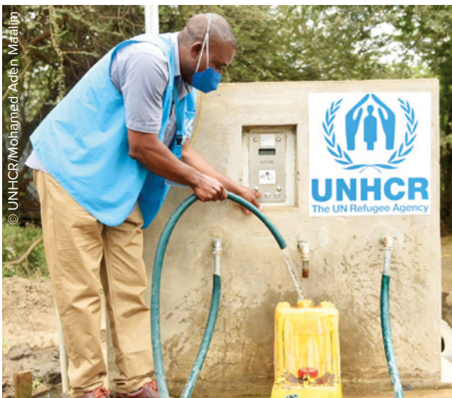
UNHCR Dadaab’s WASH staff demonstrates the use of a water ATM in Dagahaley refugee camp
