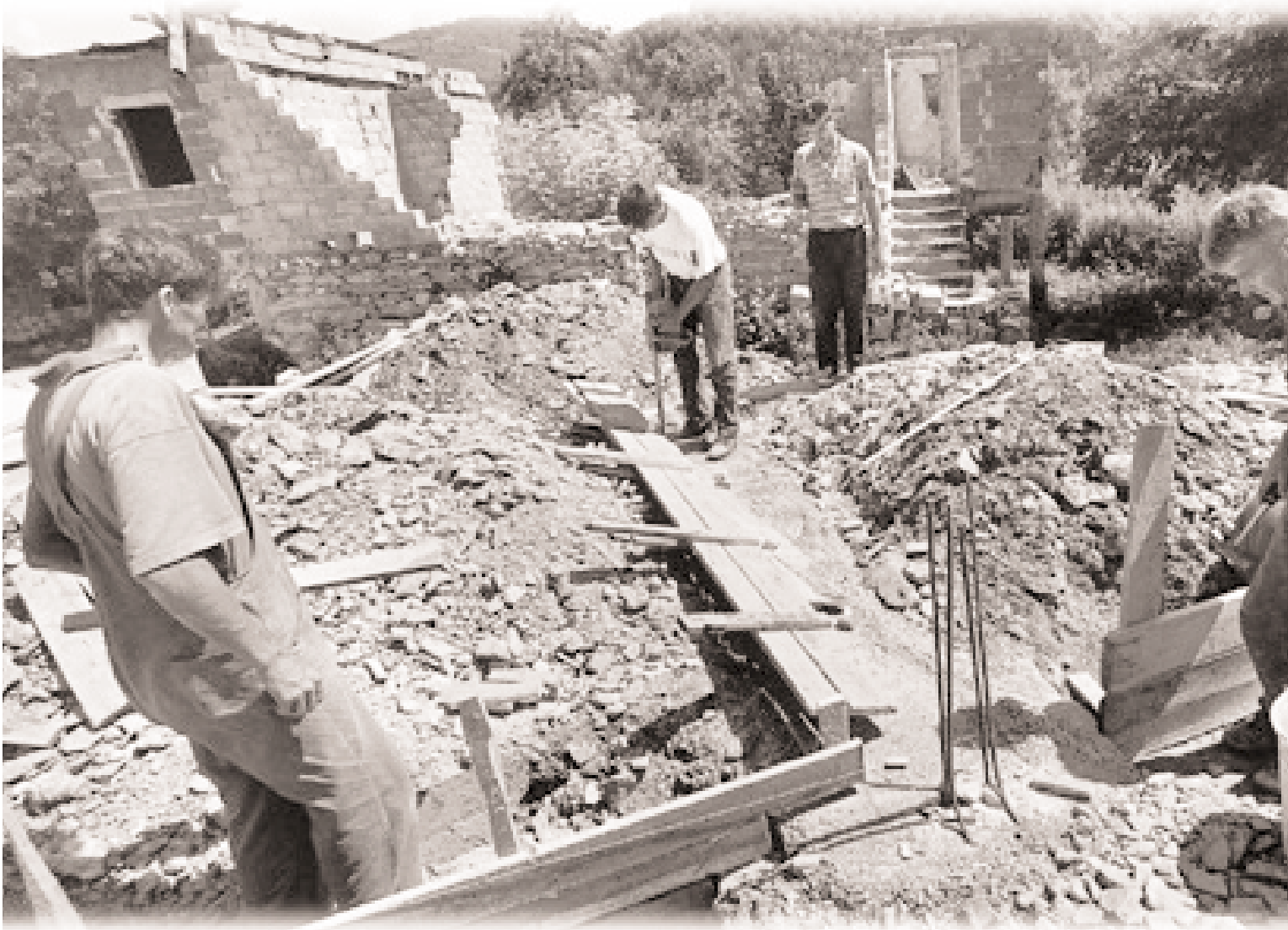
Bosnia and Herzegovina: Returnees rebuilding their house. UNHCR/R. Chalasani.
