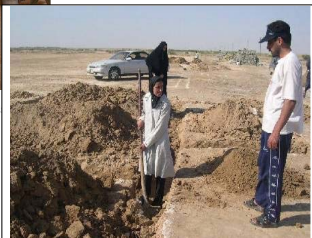
Returnees helping in the construction of shelters in southern Iraq / UNHCR
