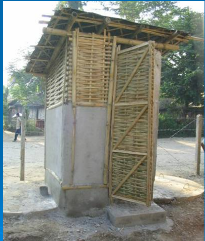
A VIP latrine
