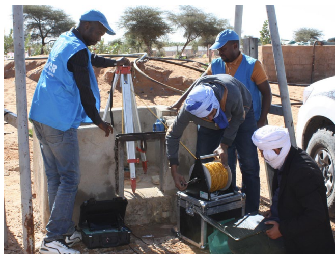
Pumping test as part of the feasibility study for the solarization of water boreholes. © UNHCR
