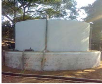
Newly constructed 45,000 liters ferro-cement tank in E-Block, NYP camp, Bangladesh
