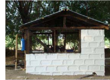
Rehabilitated pump house at borehole 3 in Dagahaley, Kenya
