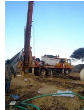
Borehole drilling in Shedder camp, Ethiopia
